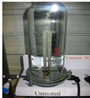
Scale buildup on heating element in untreated water
